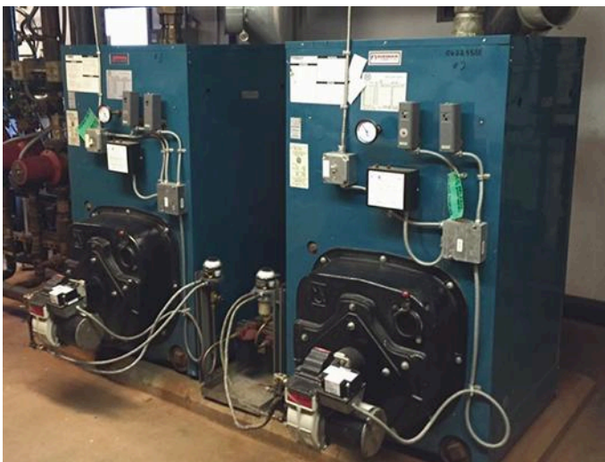
The run times for the fuel oil boilers have been dramatically reduced by the new system configuration.
