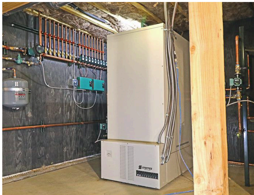
Two large Steffes electric thermal storage units, or boilers, supply the large home's 9-in. floor zones.
