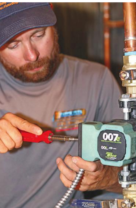
Hydronic technician Luke Drummond installs a Taco 007e circulator on each electric thermal storage unit.
