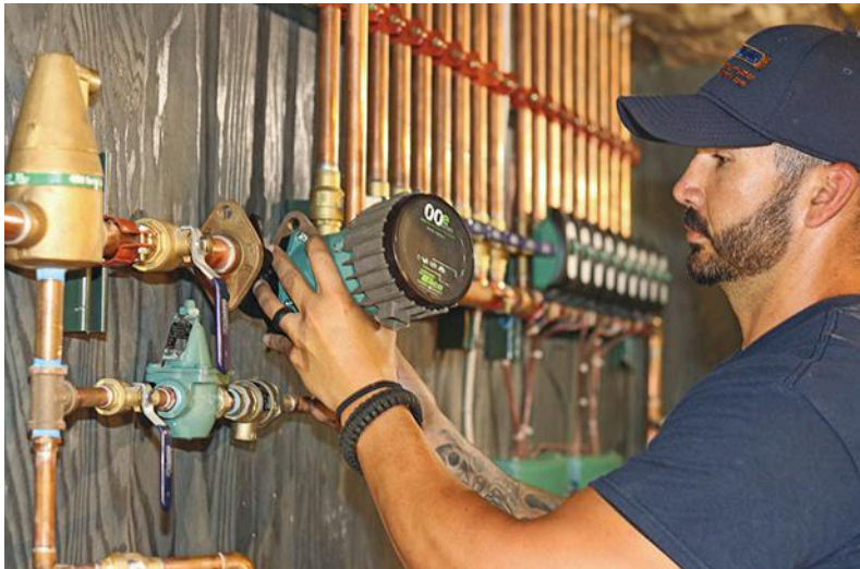
Hydronic Technician Derek Leveque installs a Taco VR3452 as the home's main system circulator.
