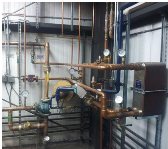
The flat plate heat exchanger (shown at the right) is connected to the primary loop to recover waste heat from the diesel generators.
