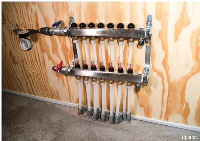
One of seven stainless steel manifolds controlling a total of 27 heating circuits throughout the Johnson Residence.
