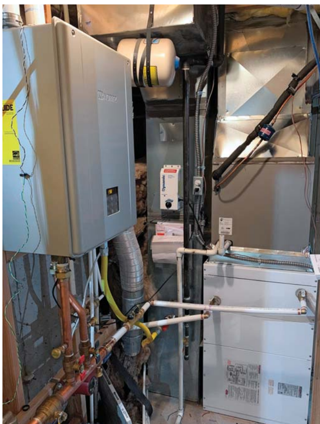
The Johnson Residence mechanical room after the installation of the new combi boiler and air handler. "The heating side works great for us. It is a lot quieter than the system that was installed before," says Gail Johnson, who added back the condenser coil from the previous setup in the mechanical room to provide cooling.
