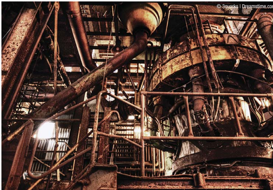
Above, an abandoned foundry.
