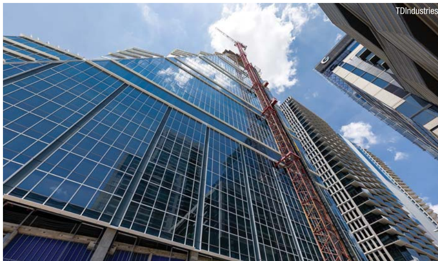
Off-site staging was a key factor in hitting crucial delivery windows.
