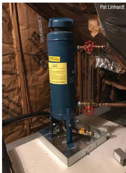
A chemical shot feeder expansion tank.
