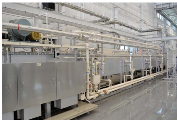
The brazing furnace.
