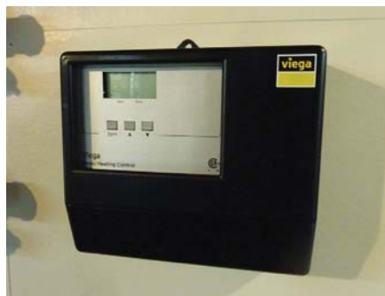
An Outdoor Reset Control from Viega.
