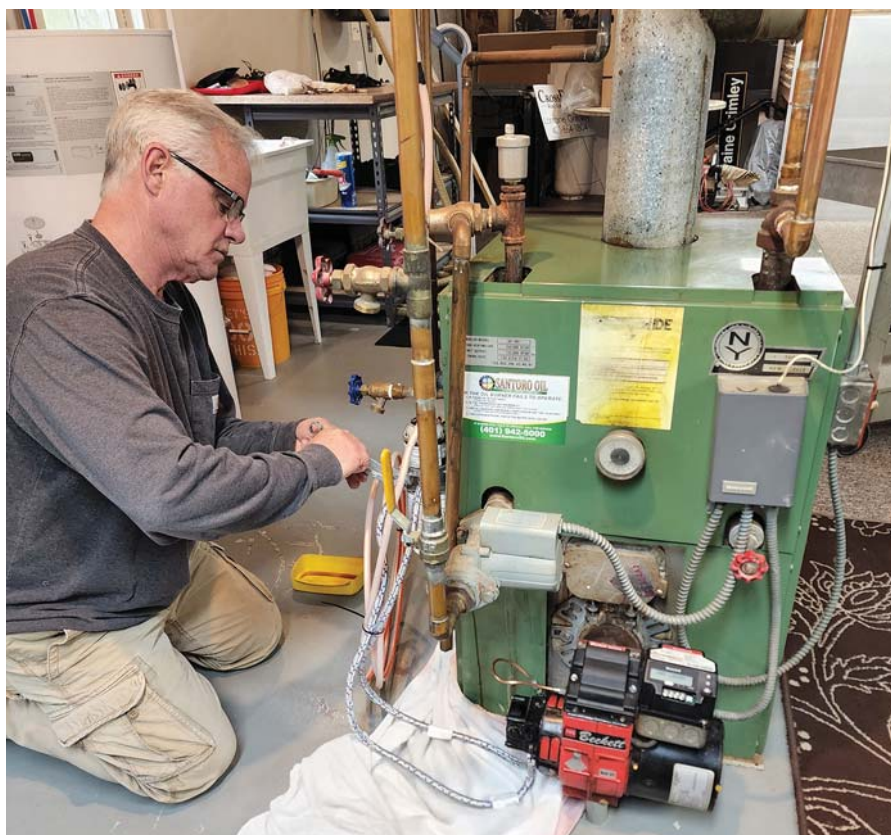
The original oil-fired boiler being uninstalled.
