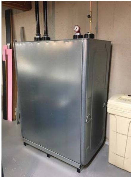
A Roth Double-Wall Oil Tank, Model DWT 1000L, with 275 Gallon Capacity.
