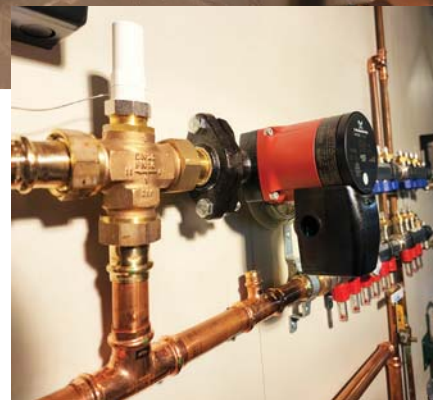
A Grundfos Mixing Station Modulating Circulator, Model 99287244 ALPHA2.
