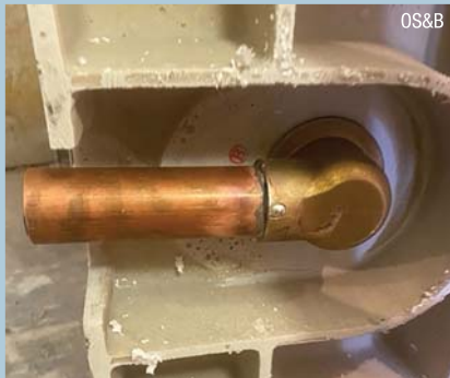
Side view of shower pan showing the side discharge shower body with brass pipe attached.
