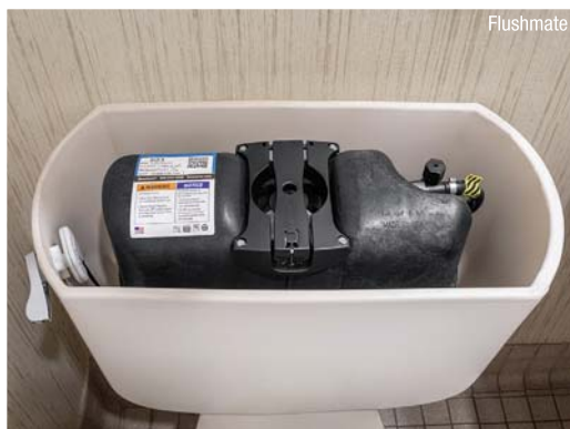
A view inside a pressure-assisted toilet tank.
