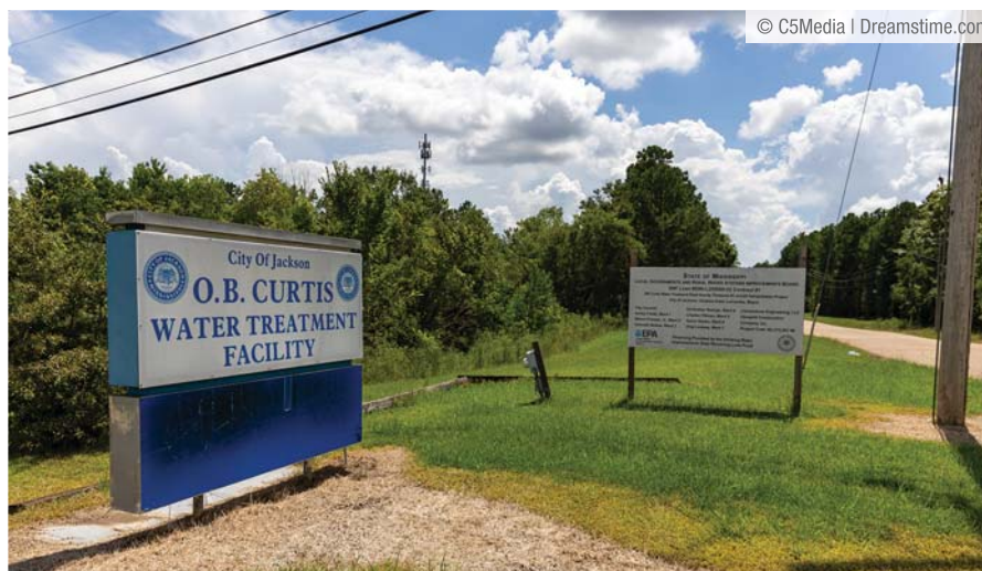
Outside the O. B. Curtis Water Treatment Facility in Jackson, MS.
