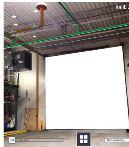
Myco using AR to image a future roof drain (brown) just left of a garage door (white).
