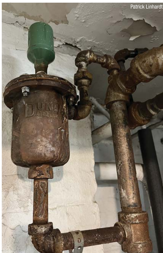
A Dunham Air Eliminator, an artifact from the early days of steam heat.
