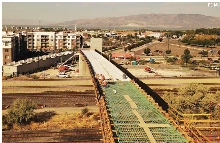
The pedestrian walkway under construction.
