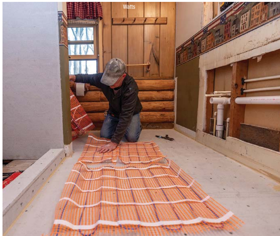
An installer laying out SunTouch radiant mats.
