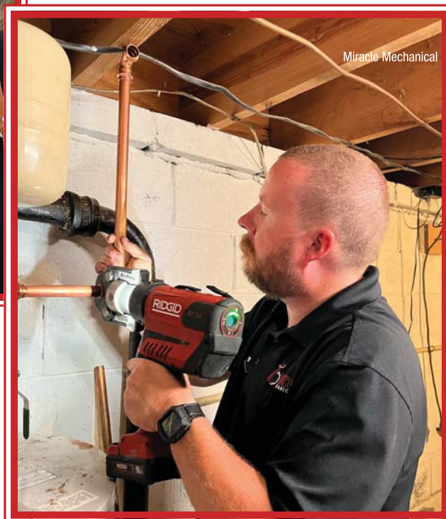
Brent Ridley works on a whole-house re-pipe project replacing corroded galvanized pipes with new copper piping and 80 lbs. of ProPress fittings donated by Viega.
