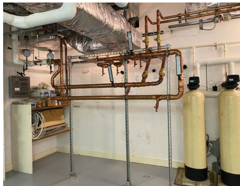
The start of the strut framework in the main house (left). The completed repipe in the main house (right).
