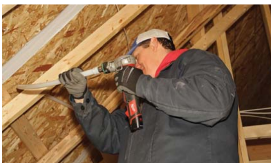
The home incorporates vaulted ceilings on the top floor which gave the installers a bit of trouble when laying out the Uponor AquaSAFE™ fire sprinkler system.
