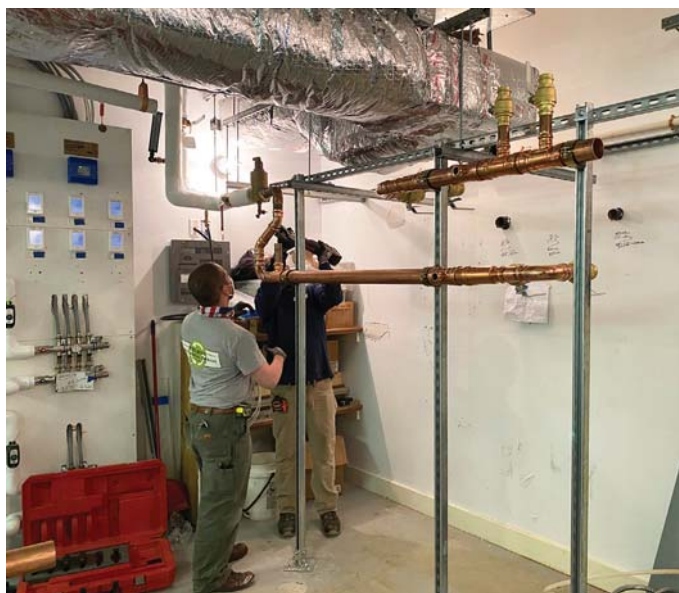
The start of the strut framework in the main house (left). The completed repipe in the main house (right).
