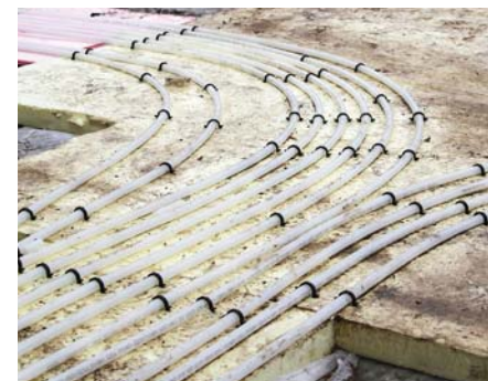
In the course of the project, Signature Mechanical installed 3,400 ft. of Wirsbo hePEX™ tubing.
