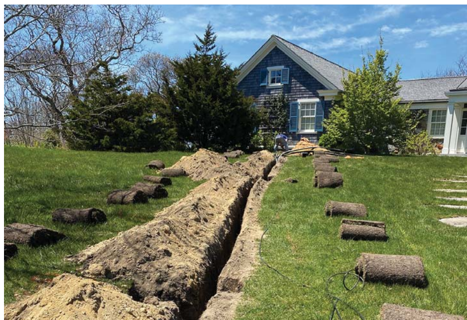
The supply return piping running from the carriage house to the main house.
