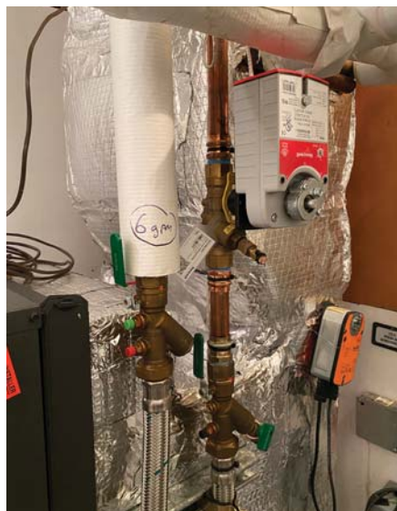
The motorized PICV ball valve in the main house mechanical room.
