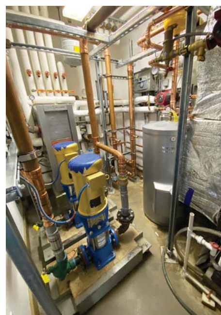
The carriage house mechanical room with the new loop pumps in place (left). The carriage house mechanical room with the supply piping connected (middle). The very crowded mechanical room in the carriage house (right).
