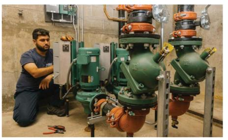
A NETE technician checks on the new Taco SKV vertical, in-line self-sensing pumps at the Greenwich Catholic School.
