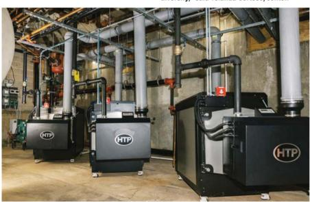
Three HTP Enduro Ti 750 MBH boilers in the mechanical room at Greenwich Catholic School.
