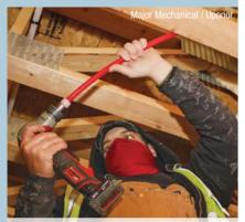
Major Mechanical installer expanding PEX pipe with the Expander Tool before inserting a fitting.
