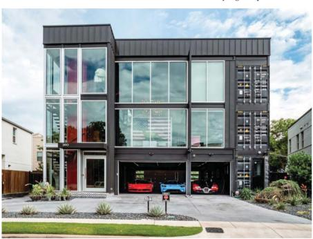
The 5,500-sq.-ft., three-story home was constructed using six 45-foot shipping containers welded to a steel-centered superstructure.
