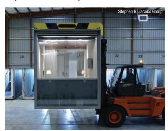
A modular bathroom unit being transported from its assembly site to a shipping area.
