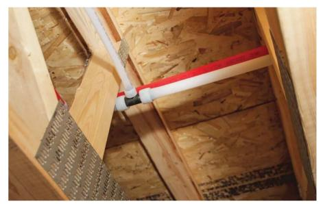
Finished PEX connections. Uponor's new kitting program provides plastic bags loaded with precise, hand-counted numbers of elbows, tees, rings and other PEX piping components to make connections like the ones shown here in a given job-site area.
