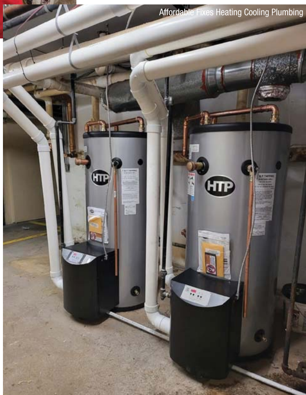
The Phoenix water heater's modulating burner operates at a five to one turndown ratio, which provides high system efficiency even during low load conditions. The heaters also comply with SCAQMD Rule 1146.2 – ultra low NOx emissions – making it eco-friendly.
