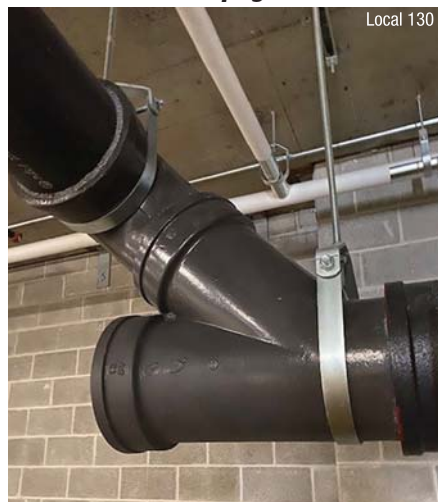
Pipe and fittings have different coating requirements.
