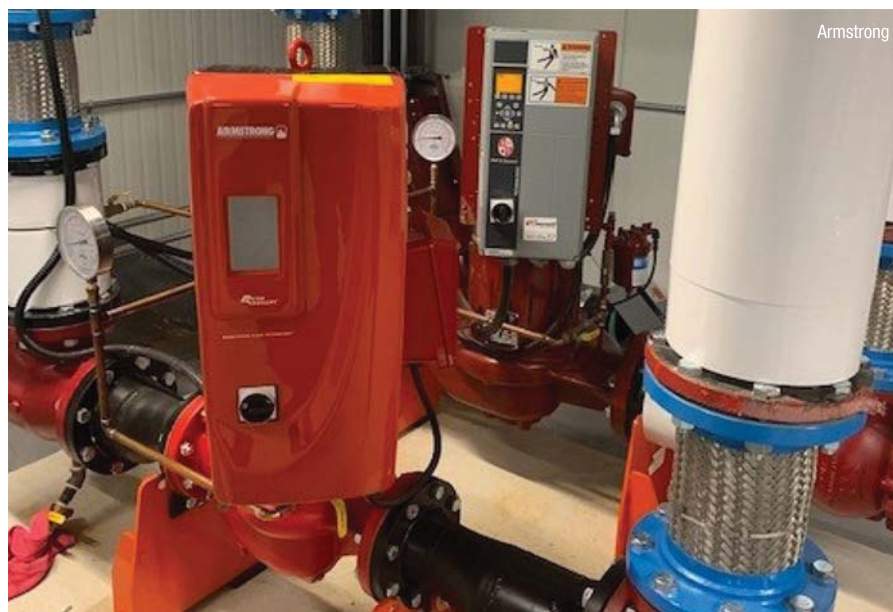
A partial view of the pipe-mounted UL 778 pumping unit
