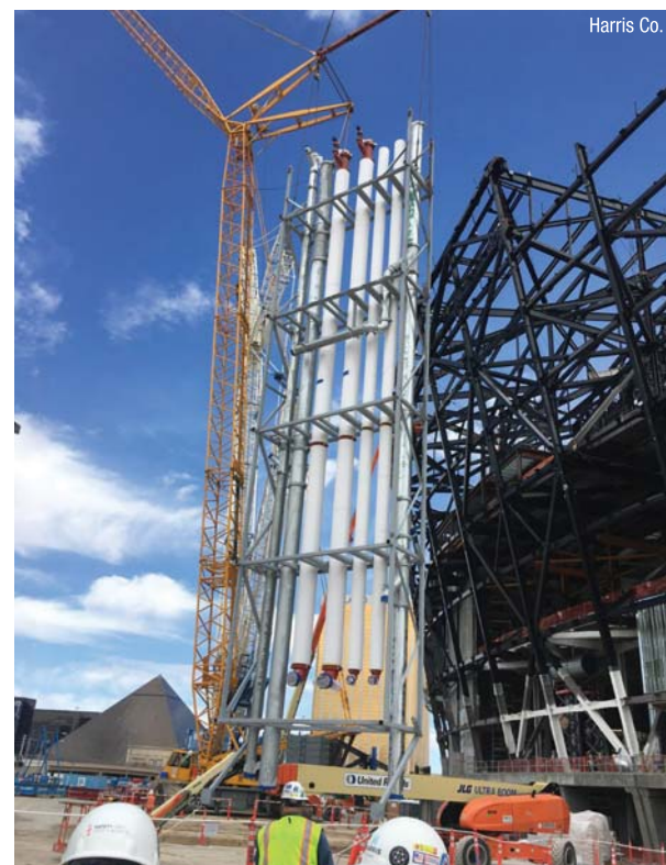
Harris Co.'s new facilities allow for very large prefabricated assemblies.
