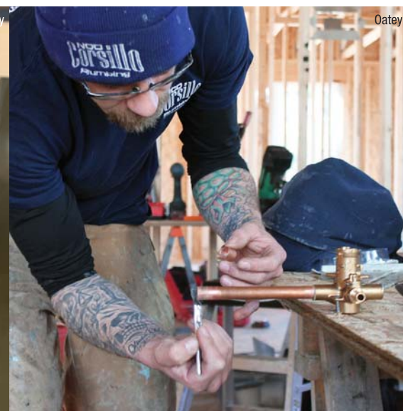
(Left) A tech soldering a copper joint. (Right) A technician applies flux to the end of a piece of pipe.
