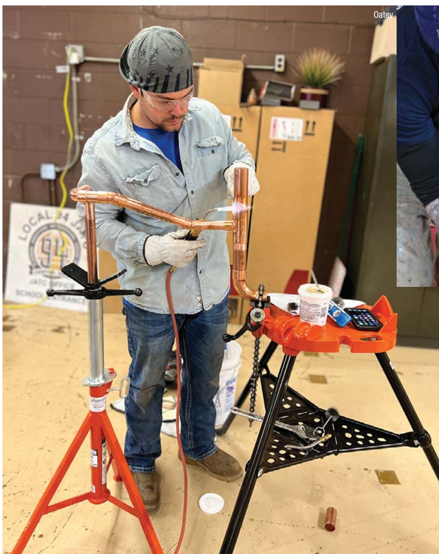
(Left) A tech soldering a copper joint. (Right) A technician applies flux to the end of a piece of pipe.
