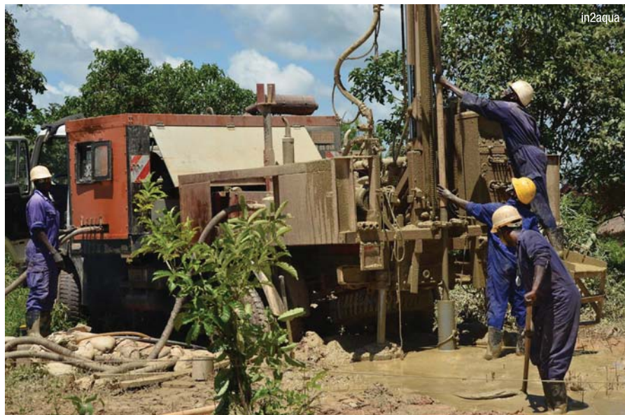
A well building team used a truck-mounted drill rig made by Atlas Corp.
