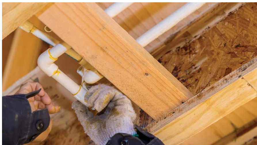
A technician fitting pieces of CPVC pipe together with solvent welds.
