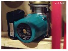
The addition of a recirculation pump (from Wilo) means instant hot water delivered to the end use point.
