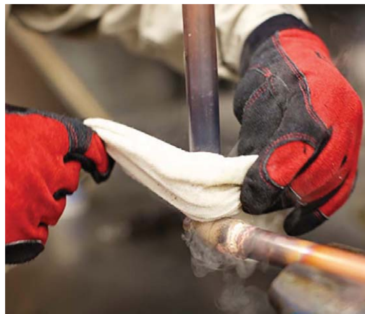
Once the brazing is completed, it's important to remove all flux residue because flux is alkaline and could corrode the base material.
