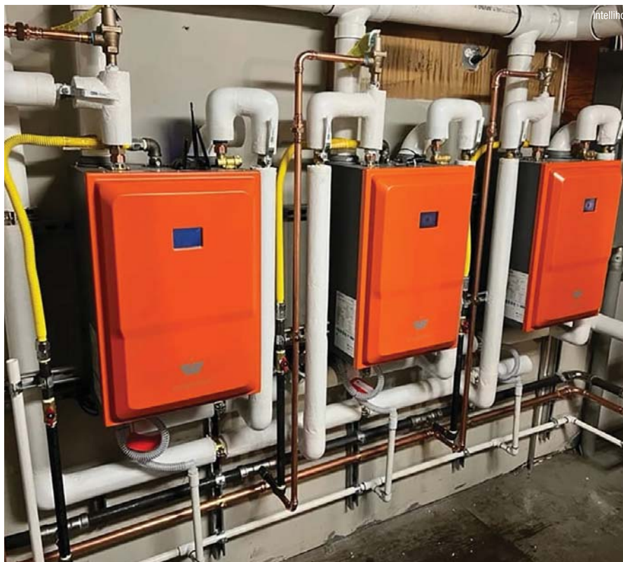
Intellihot has units that can be installed in series to deliver the high capacities commercial customers require.
