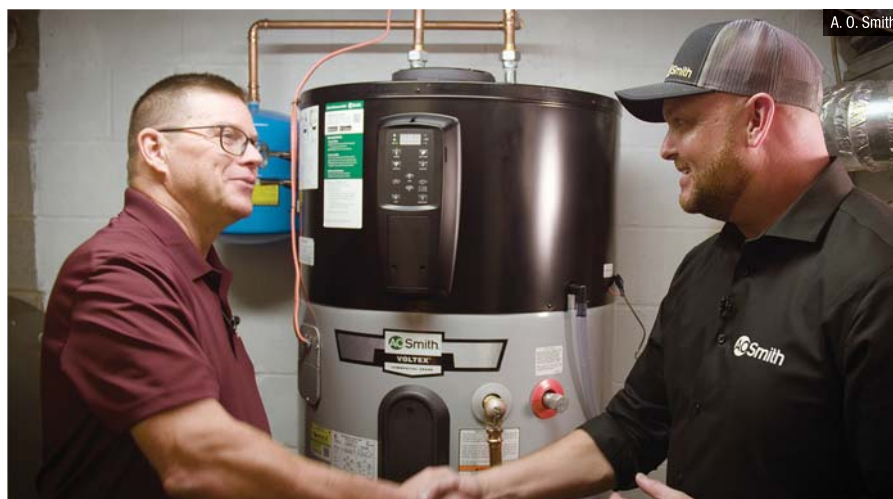
Gerry Winset of A.O. Smith (right) shakes hands with Carl (left), a tech working with W. L. Staton Plumbing, Cooling & Heating, in front of a Voltex hybrid electric heat pump water heater.
