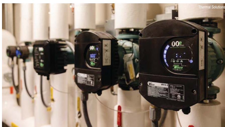
Five Taco 00e circs of varying size govern the zones and a larger Taco 1915e serves the primary loop.
