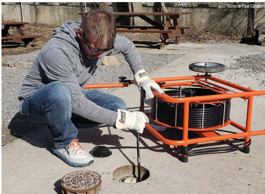
A service technician cleans a drain.
