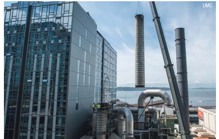
The Enwave smokestack replacement job.
