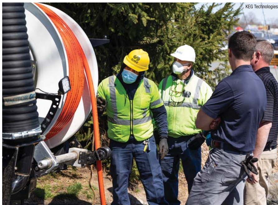
Workers wearing their PPE at the vacuum truck. To prevent free spooling the nozzle up the line and losing control, use a nozzle skid and hold the nozzle back.
