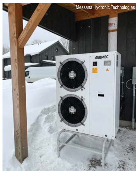
The 5-ton Aermec heat pump that is the heart of the system.
