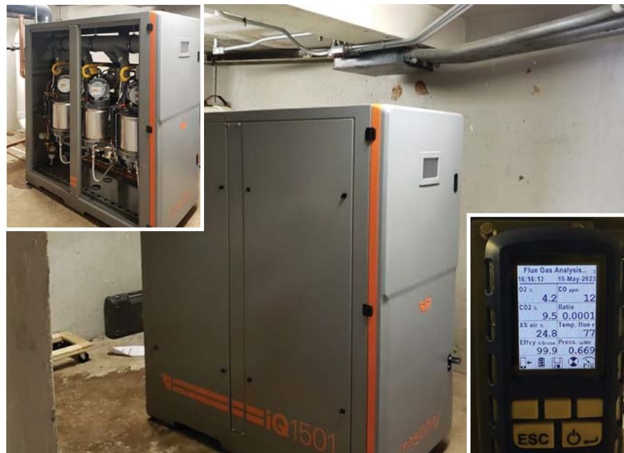
The Intellihot iQ1501, shipped from F.W. Webb, installed. (Top inset) Intellihot iQ1501 with doors removed. (Bottom inset) Efficiency meter showing the iQ1501 operating at 99.9%.
