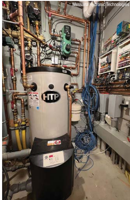
The system also includes an HTP Phoenix high-efficiency water heater as a backup for the heating side of the house. The Phoenix has a 96 percent thermal efficiency rating.
