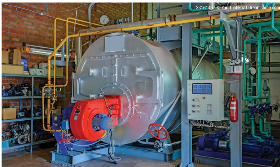
A steam boiler on gas fuel.
