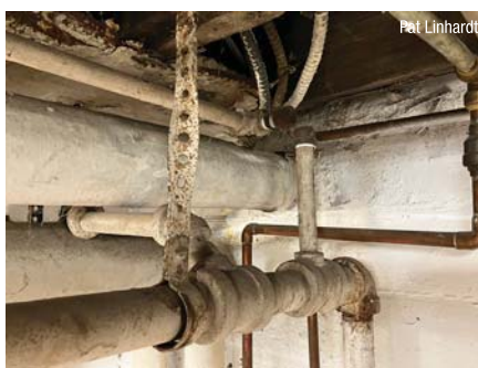
Originally, there was a trap between the two 1/2" caps. Now, there isn't a path for the air from the end of the steam mains to get out of the way of the steam.
