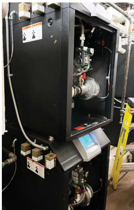
One of the Elite boilers with its service cover off.
