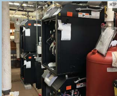
A view of the new mechanical room showing two of the four new Elite XL boilers.
