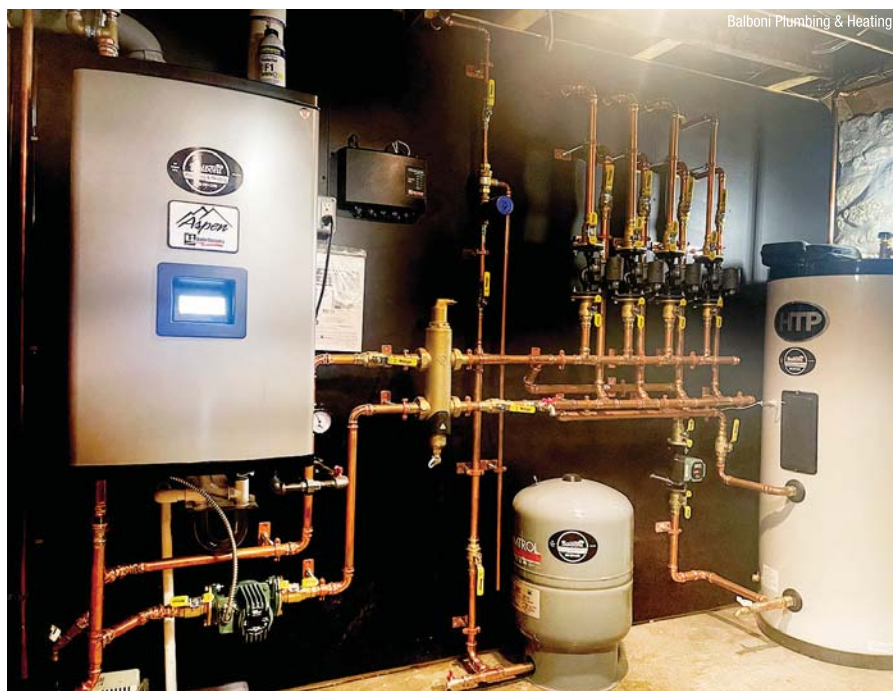
The new hydronic system serves cast iron radiators from the 1800s.
