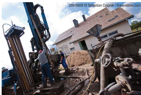
Two workmen drilling a residential geothermal field.
