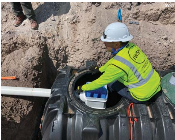
The mound systems are able to treat wastewater from the homes as well as eliminate the leach line ponding that had become a common occurrence.
