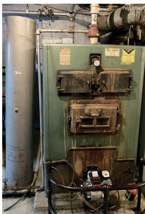
There is a weighted check valve in the supply main visible at the top of the picture, which was common for mid-century hot water jobs.
