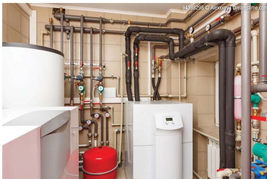
Household boiler room with heat pump, storage tank and circulators.
