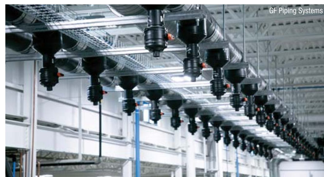
COOL-FIT Pre-insulated Piping from GF Piping Systems provides leak-free, maintenance-free cooling loops at Tree House Brewing's Charlton facility. Insulation under factory conditions improves efficiency and simplified the installation process.
