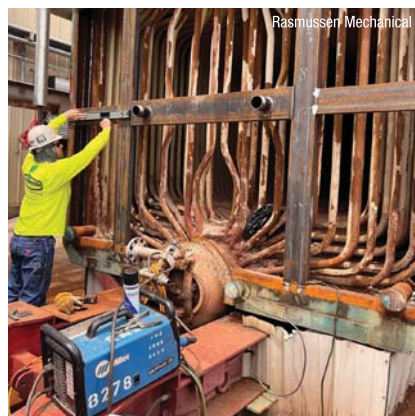
Part of the rear wall rebuild about midway through with support beams in place.
