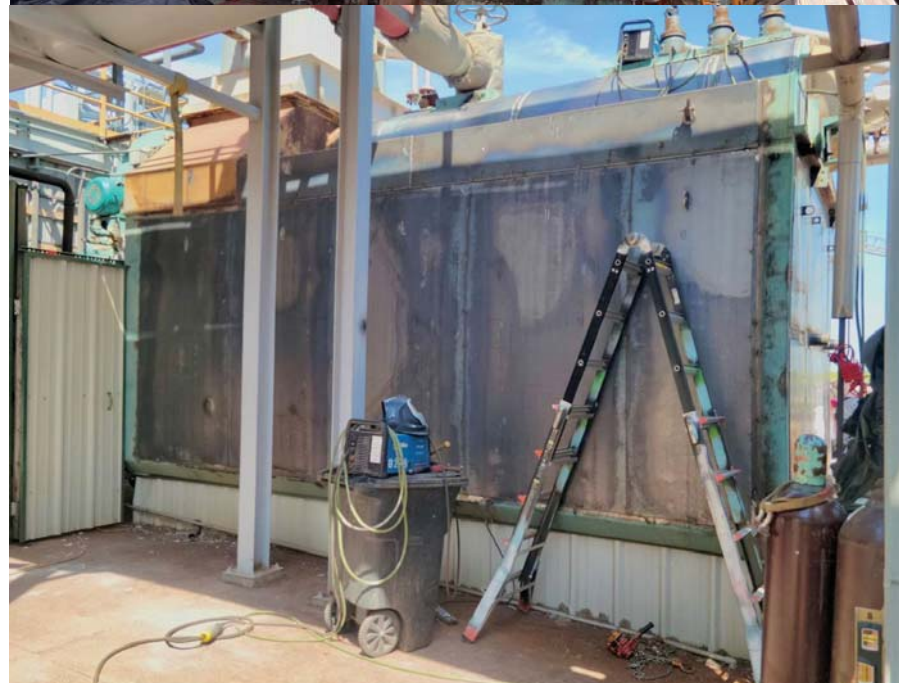
The rear wall after installing new insulation, a new wall and exterior supports.
