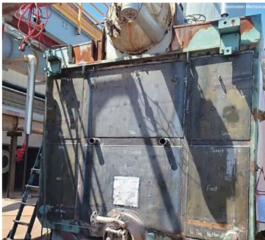
After installing the insulation and new wall, but before installing the exterior support beams.
