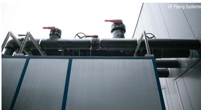
The thermal efficiency of COOL-FIT Pre-insulated Piping ensures consistent temperatures for chilled glycol throughout the cooling loops at Tree House Charlton, even with the facility's chillers located outside.
