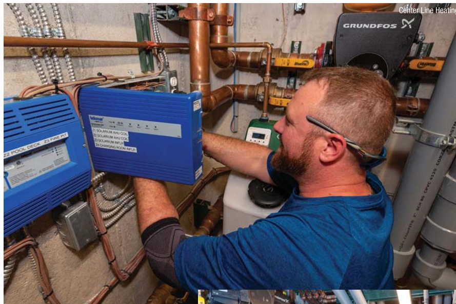
Landis, Center Line installer, wires a tekmar switching relay.
