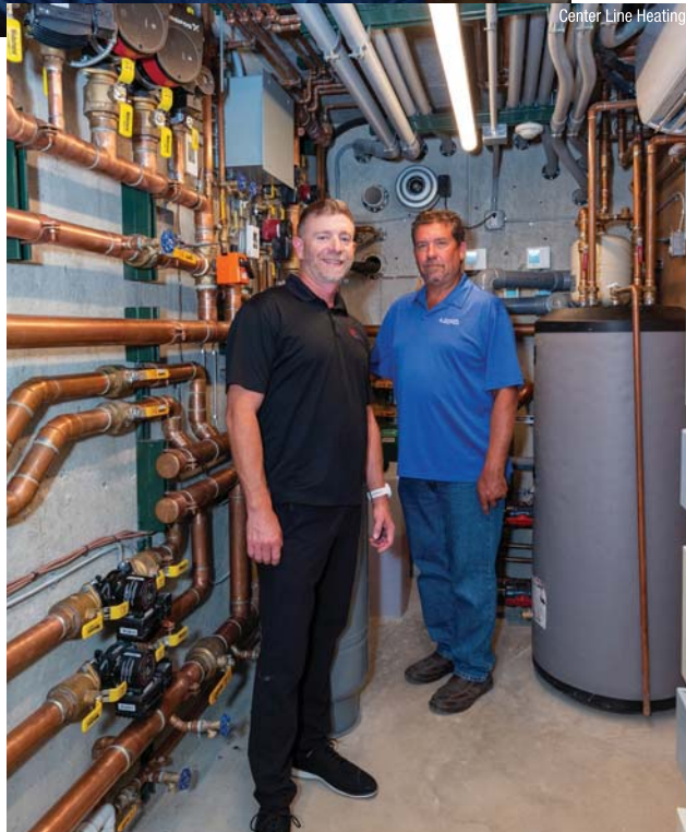
Armstrong (left) and Gillette, in the mechanical room below the terraces.
