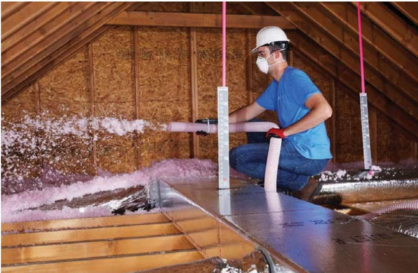
Ductwork in the attic can be easily accessed and inspected.
